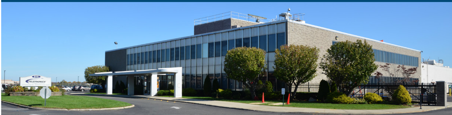
Telephonics Corporate Headquarters
